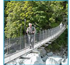
Kiwi swing bridge
